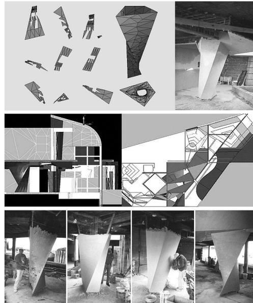
Fig.2 Unfolding NURBS surfaces and construction CHIARELLA y ASOC - Lamperti & Cia - Paraná 2001
