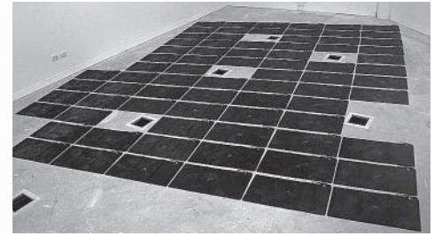
sensor technologies in furnishings, surfaces and pre-fabricated building materials (Figure 4) - facilitate localised sensate regions and unobtrusive (wireless) distributed networks for data collection.
