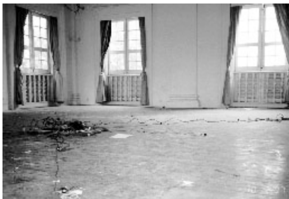
Figure 7 Interior view of Salon room
