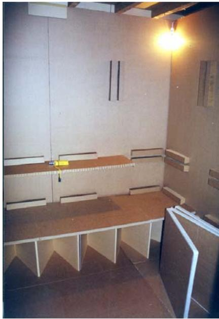
*Figure 6. Interior of shelter with bed and shelf. All made from paper honeycomb board (Koh, Leng & Teo).*
