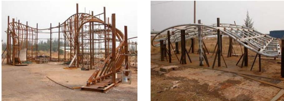
*Figure 19. Testing fabrication of the free-form structure*
