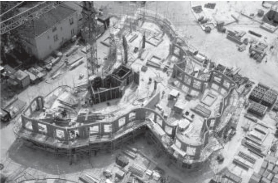
In Gehry's project in Düsseldorf (*Zollhof Towers*), the undulating forms of the load-bearing external wall panels, made of reinforced concrete, were produced using blocks of lightweight polystyrene (Styrofoam), which were shaped in CATIA and were CNC milled (figures 3.17a–f) to produce 355 different curved molds that became the forms for the casting of the concrete.<sup>5</sup>
