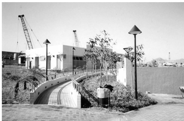
Figure 4. Existing public toilet.
