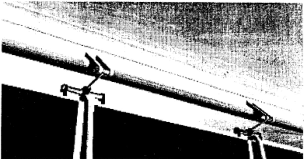
Fig. 12 Glazing to roof movement joint
