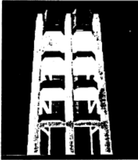
Fig. 6 Alternative masonry loadbearing columns
