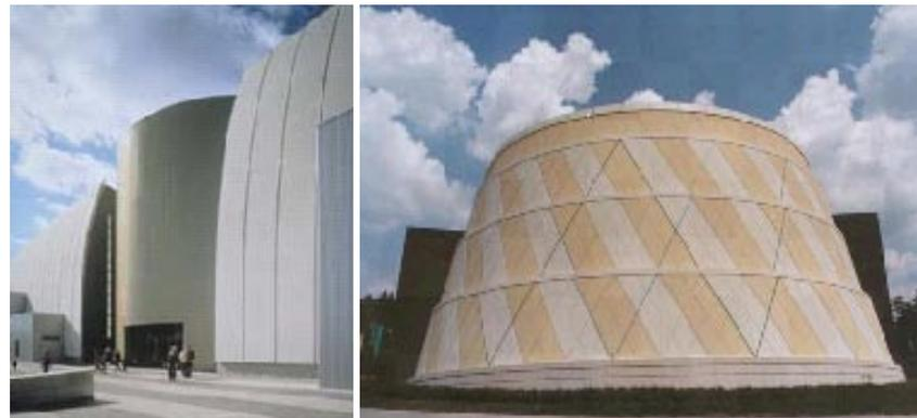
Figure 4: Some complex forms and detailing with precast concrete
