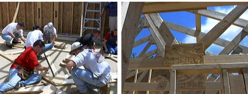
Figure 7. On-site truss fabrication and joint detail
