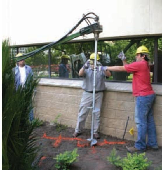
Figure 12. Helical Anchor Installation.
