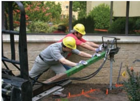
Figure 13. Driving the Anchors to Achieve the Target Torque.
