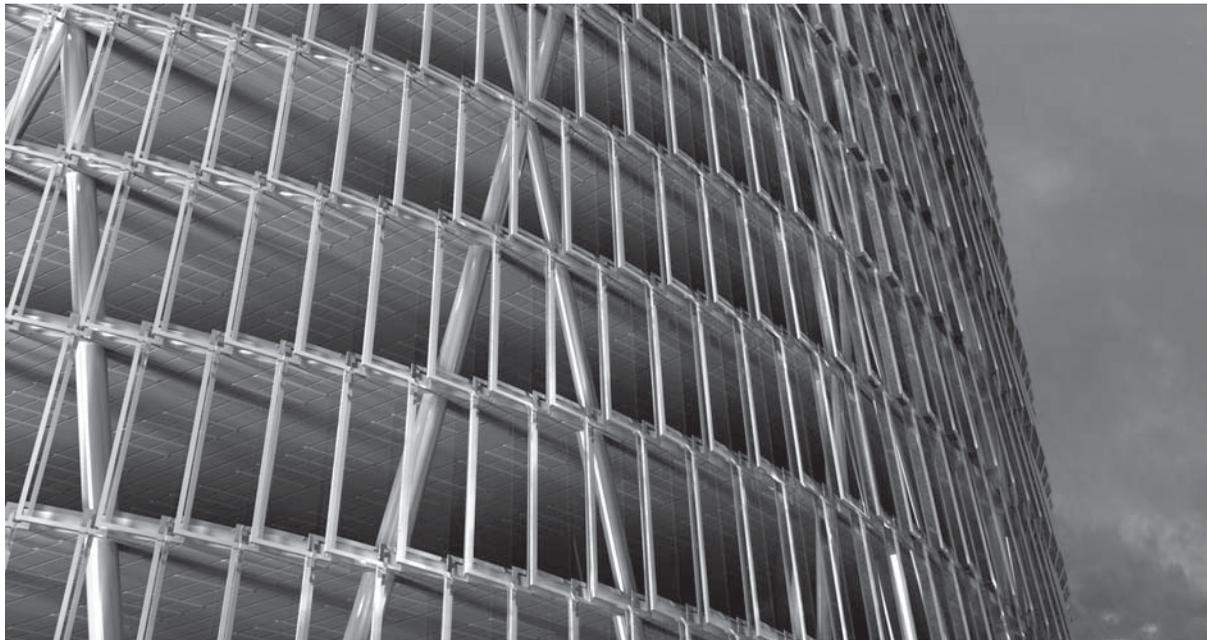
**FIGURE 12** Final configuration of the shingle panels on the building surface.
