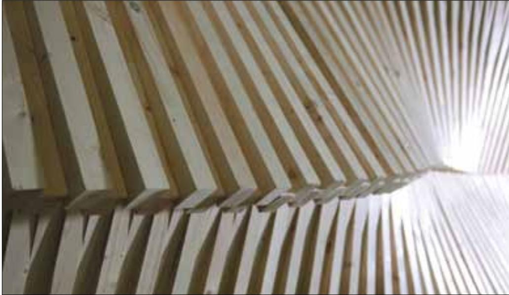
Figure 4 Smooth Surface Ideal for Water Drainage in Wood Grain Direction
