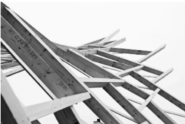
Figure 14. Detail of Lamella joint in 1:1 demonstrator in Oslo
