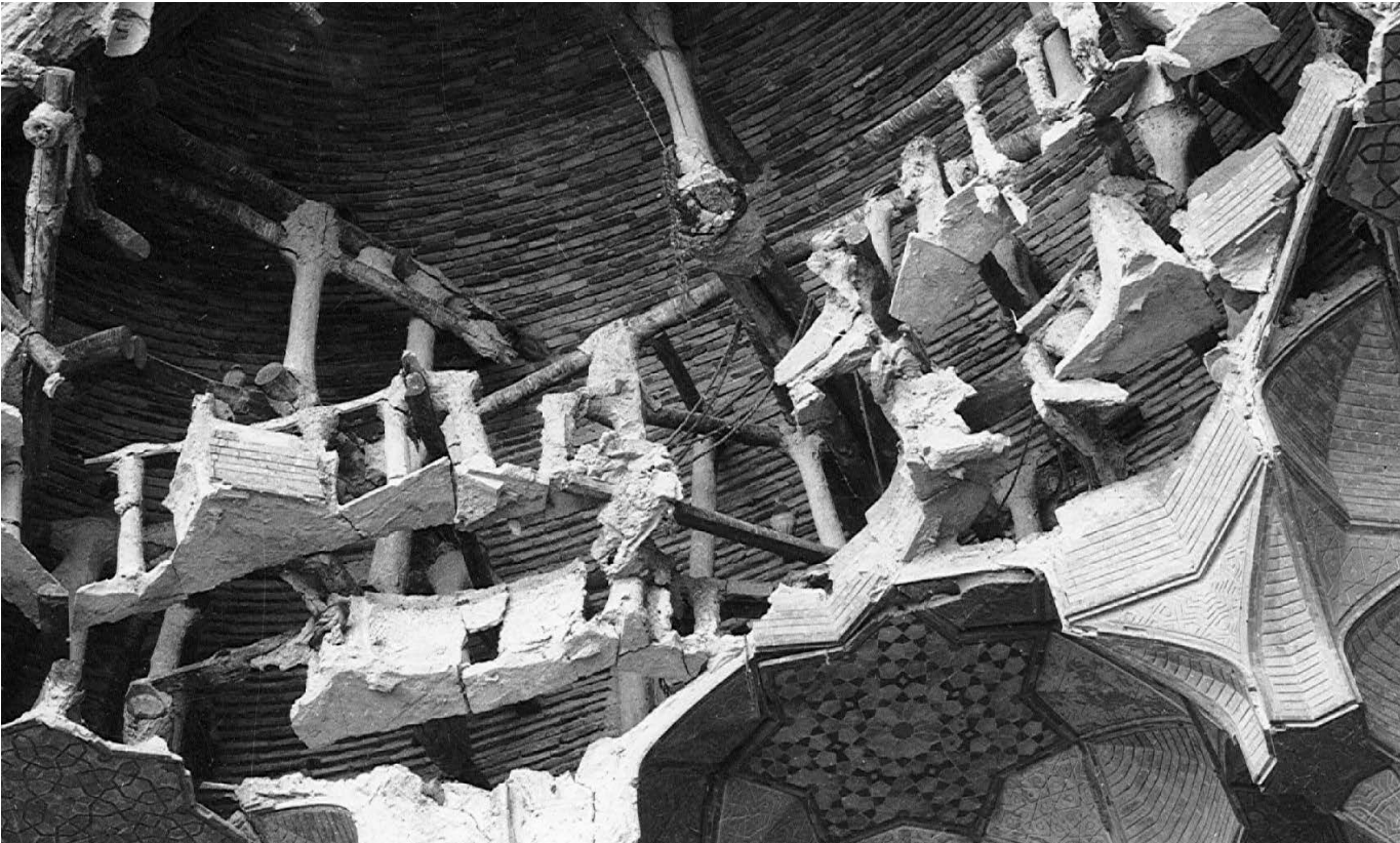
1 Muqarnas under reconstruction in Yazd, Iran (Aga Khan Archive, Harvard Fine Arts Library)
