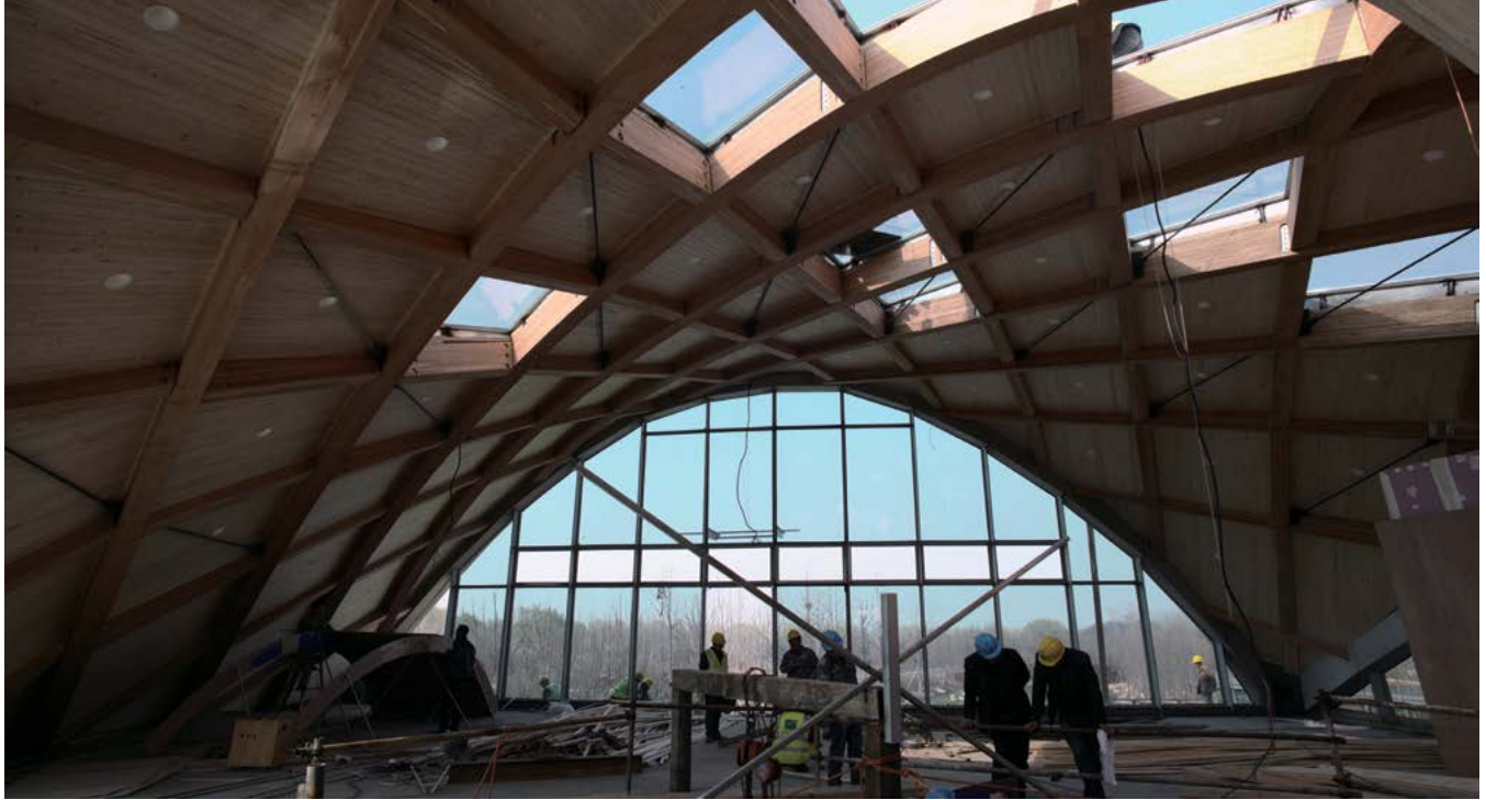
22 Interior View of Timber Shell System.
