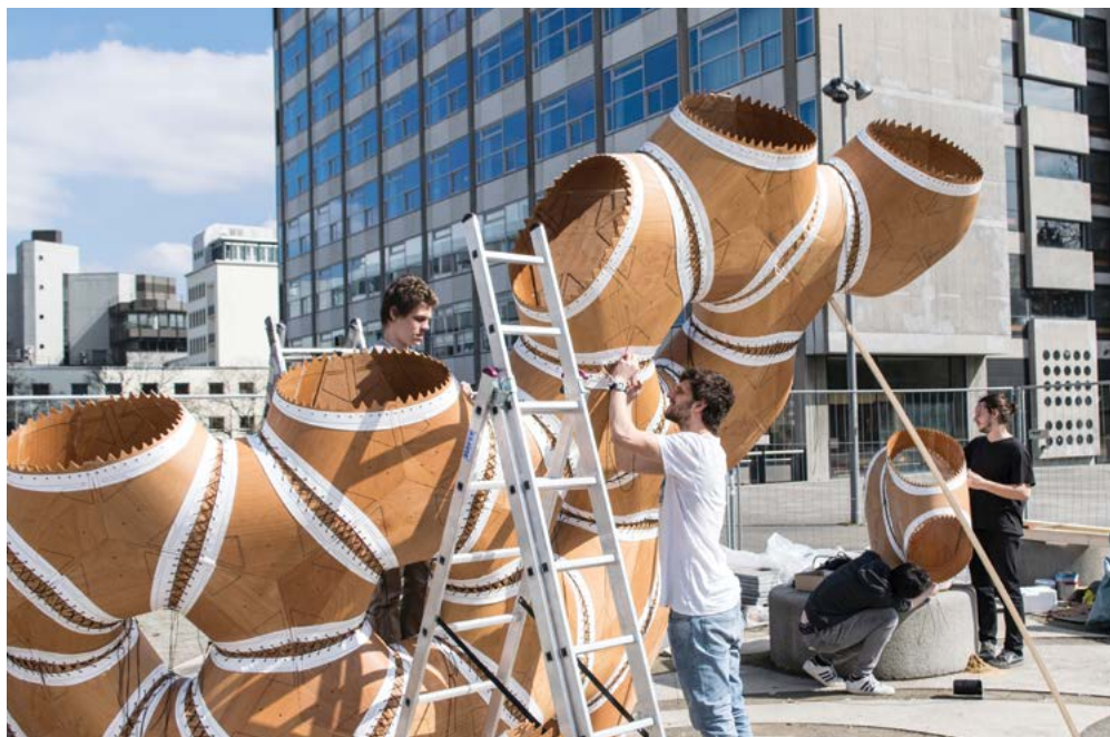
10 Assembly process of the demonstrator. The lacing connection's rigidity allowed the cantilevering of segments during the construction.
