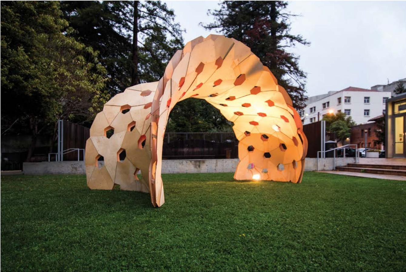
18 View of the Bend9 structure assembled out of 3 mm thin birch plywood in the courtyard at UC Berkeley's College of Environmental Design (CED).
