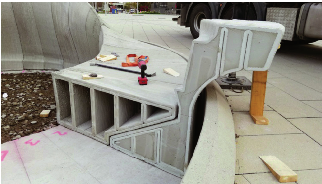
6 Sideway assembled components of the 3D printed concrete house (Carra and Stabile 2018)
