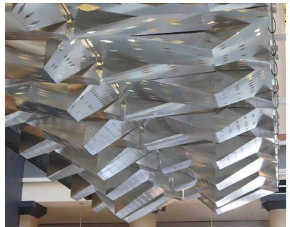
**Figure 3.** Prototype, full scale. Laser cut aluminum.
