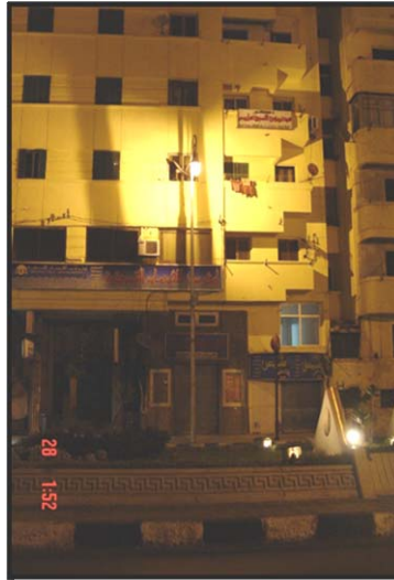
Figure 9: Façade with the lighting fixture posted on front of it (case study 2).
