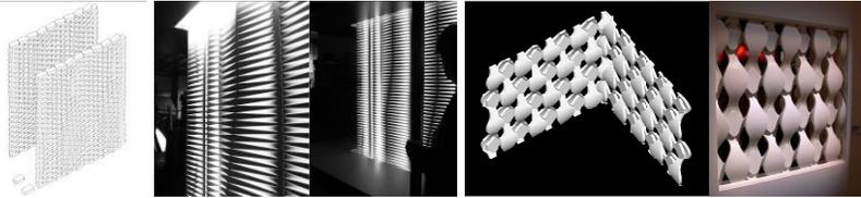
*Figures 29-33.* 29: a brick wall, with bricks rotated (using an algorithmic process) to create openings in the wall; 30-31: metal-panel wall, fabricated by Milgo-Bufkin; 32: model of "weaving wall" showing a corner condition; 33: Corian mock-up of "weaving wall" (displayed at SIGGRAPH 2008, photograph by Lira Nikolovska).
