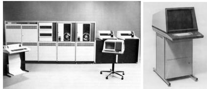
*Figures 1,2.* "Computer Room", mid 1980's, show Digital Equipment Corp's VAX mini-computer, including CPU, disk drives, backup tapes, printer, and console; Tektronix 4014 terminal "green screen" (with thumbwheels just to the right of the keyboard).
