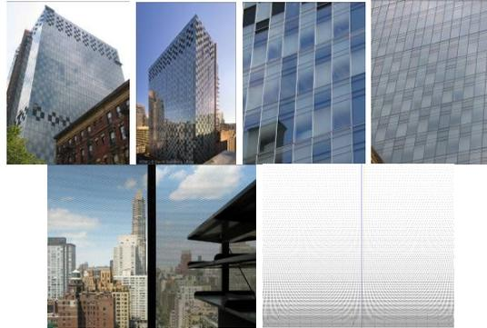
*Figures 18-23.* 18-19: photographs of the tower, showing the visual effect of the fritted glass; 20-21: close-up views of this effect; 22: an interior view, showing the glass panel at the aisle bay on the left and the glass panel at the equipment bay on the right; 23: an example of the frit pattern, showing the vertical centerline and the change in both size and spacing of the frit dots..
