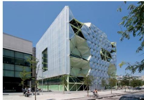
*Figure 8.* Media ICT building in Barcelona, by Enric Ruiz-Geli, features a dynamic facade made of “breathing” ETFE air cushions.
