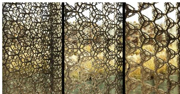
*Figure 4. Tessellate adaptive façade system designed by ABI in collaboration with Zahner Metals.*
