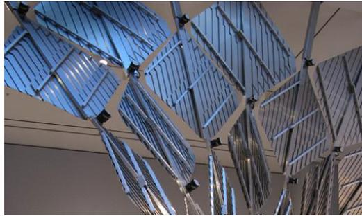
*Figure 5. Strata adaptive shading system designed by ABI in collaboration with Zahner Metals.*
