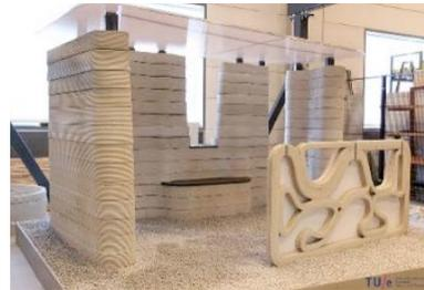
Figure 3. 3D concrete printed pavilion
