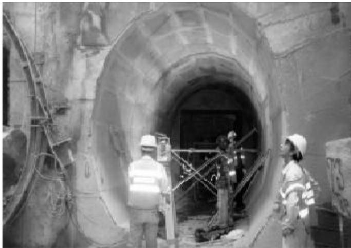
*Figure 12. Hand-mining excavation of adit for emergency use*
