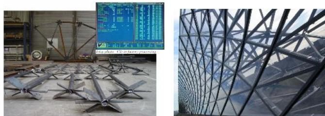
*Fig. 06 3d steel lattice model and its corresponding execution*
