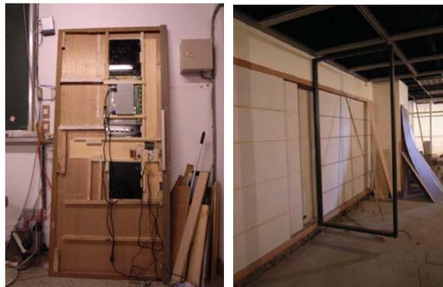
Figure 4. Left: A full-scale physical prototype of interactive wall modules. Right: The interactive moving wall system is under construction in the live-in laboratory.
