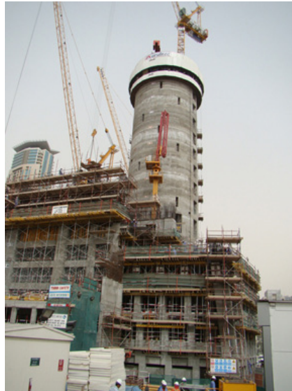
Figure 2. Dubai Infinity Tower under construction (May 2009).
