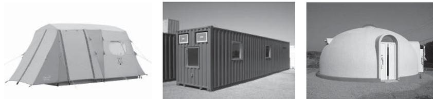
Figure 1. Lightweight structural type: (a) tensile, (b) frame and panel, (c) surface.
