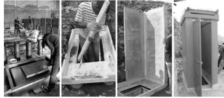
Figure 1. Application and production process used to solve a real-world sanitation problem utilising local resources and labour (2010).
