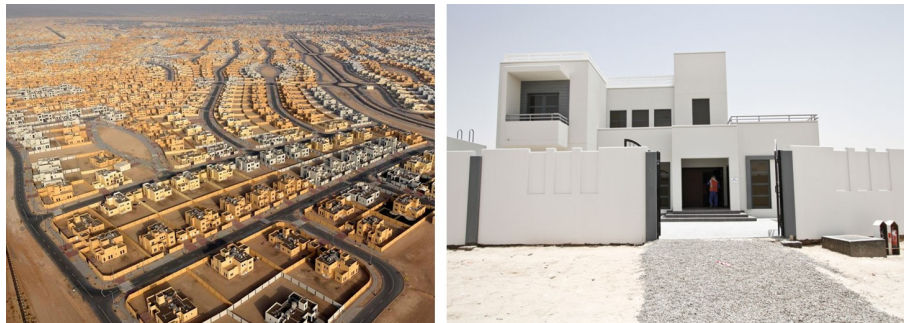
Figure 1. Images from Al-Falah housing project showing an aerial view of the site, and one of the single family houses by the company Gulf Precast (Source: Gulf Precast 2017).
