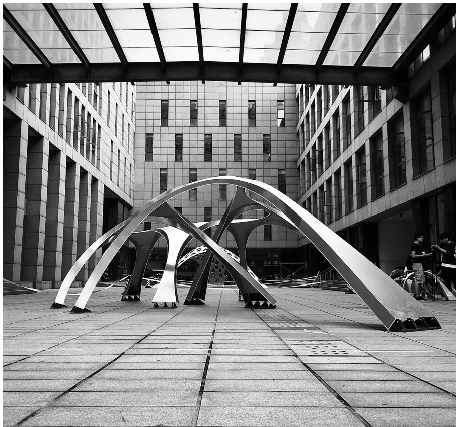
Figure 1. A Full-scale Long-span Pavilion built with the structure concept .
