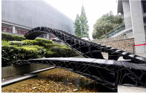
Figure 1. first 3D printed modified plastic pedestrian bridge in China.
