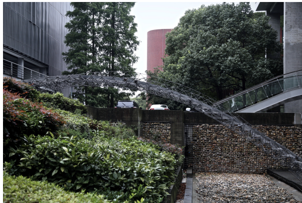
Figure 2. 3d printed metal bridge.
