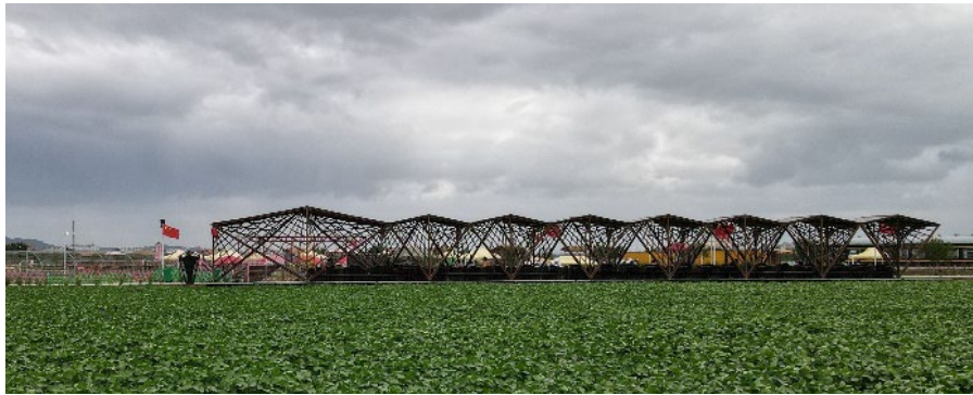
Figure. 1. The bamboo pavilion "Diecui Gallery"
