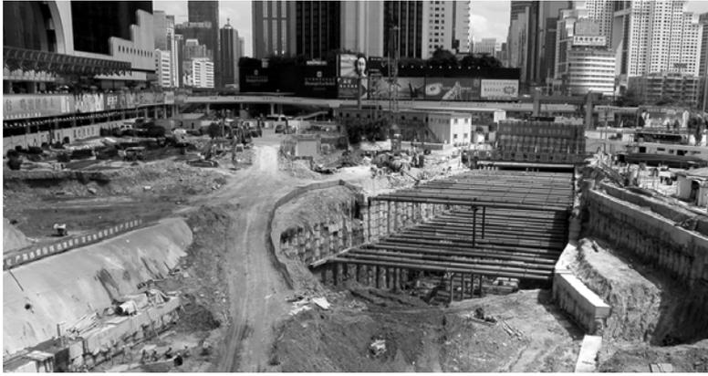
**Figure 4 Cut and Cover Execution of a Subway Station in Shenzhen (China)**
