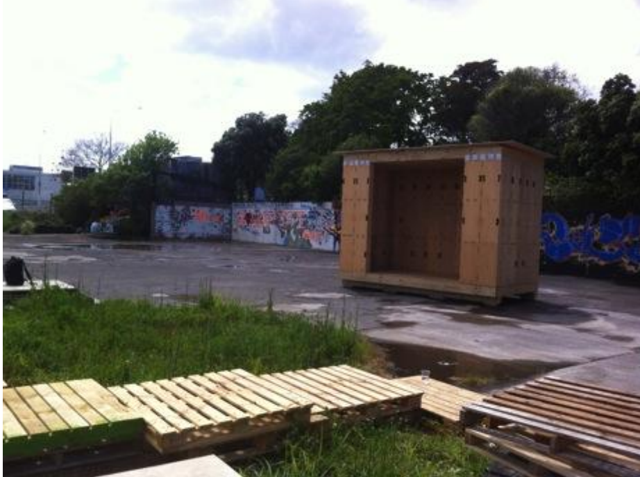
Fig. 8. Finish unit as site beings to exhibit signs of vandalism
