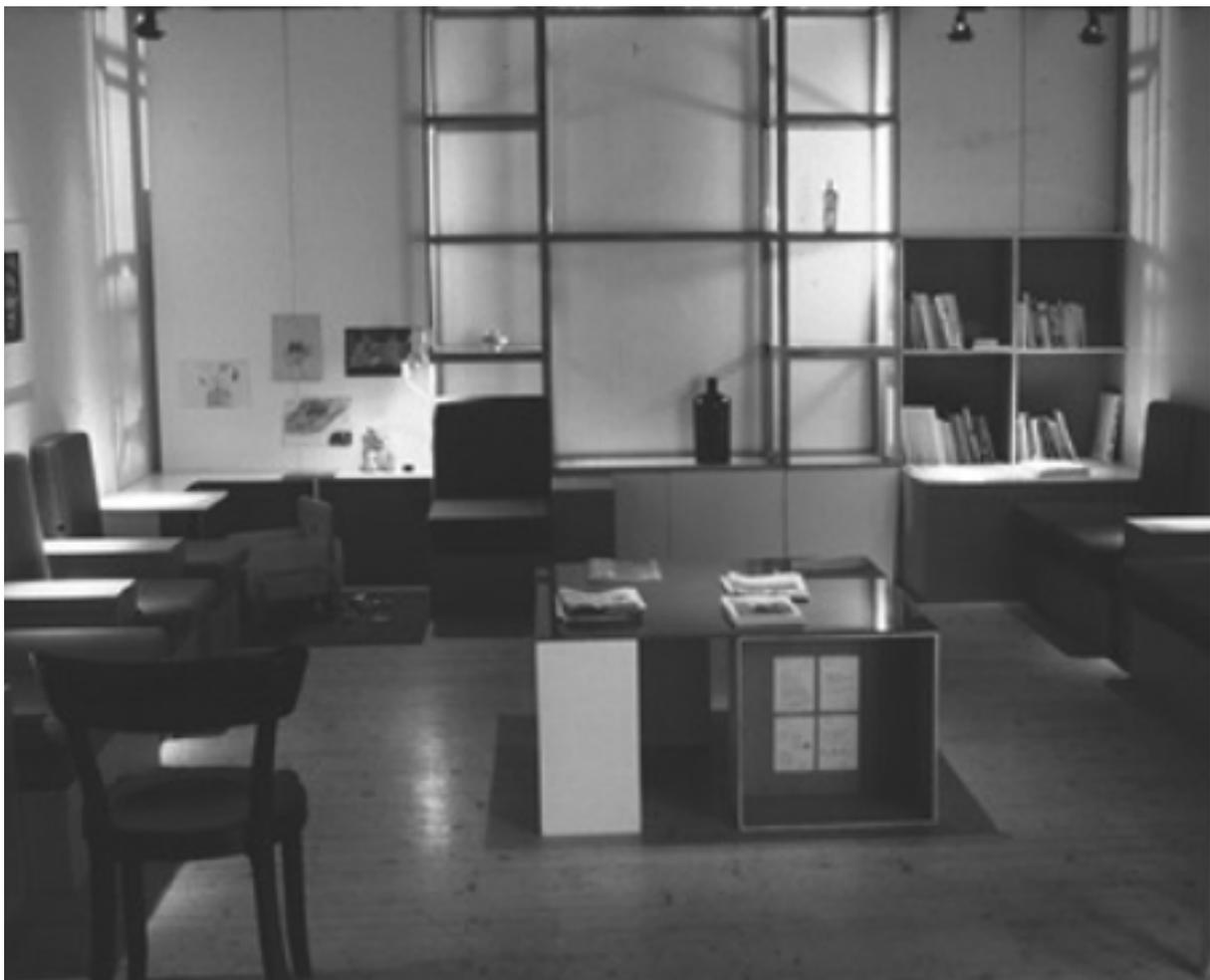
Fig. 5 A steel construction may be used to enlarge an existing window.
