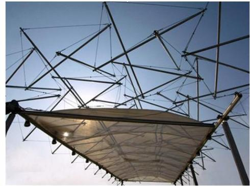
addressed (Figure 2). The same software application can generate the pre-stressed and the loaded configuration of such networks.
