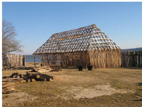
Figure 5 Mockup Structure at Jamestown developed by Bill Kelso's team.
