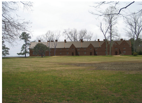
Figure 2 Statehouse digital reconstruction superimposed on foundation wall.
