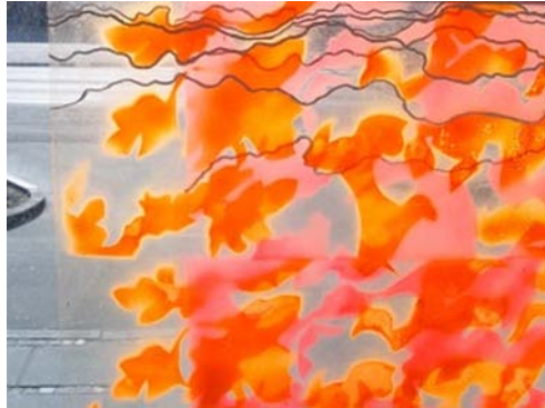
Figure 4 Constructions in EX 1, Ornamentation in glass facade imitating red color pigment and electrical conduits in PEC solar cells to illustrate how solar cell technology can effect daylight in the façades and interiors.
