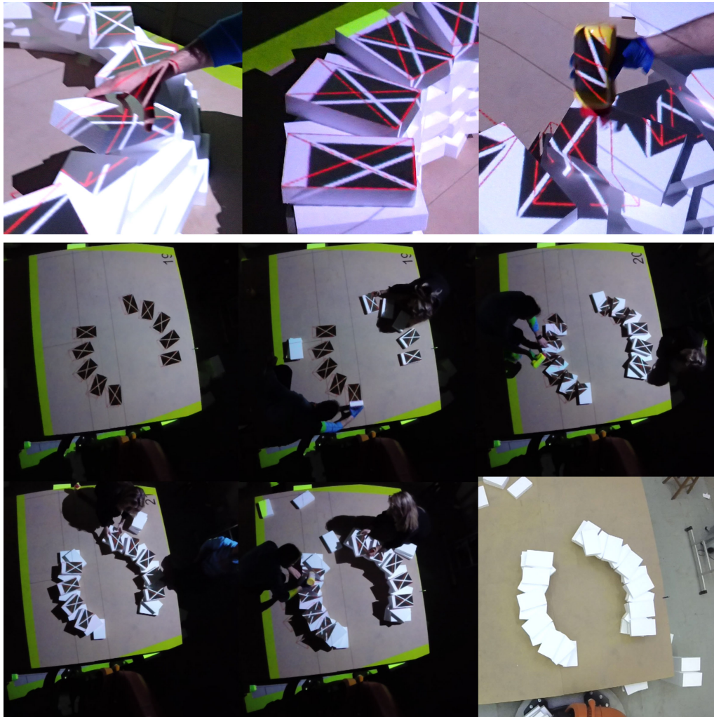
Figure 6 In the top row: (left) the dark crossed rectangle indicating the position to laid the brick; (center) the bright crossed rectangle matching the upper surface of bricks confirms that they were laid right; (right) the portion of the dark crossed rectangle (the position of the upper brick) over the laid brick indicates the area to put the glue. In the bottom: a sequence of the manual process of assembly the structure with the aid of the video projection technique.
