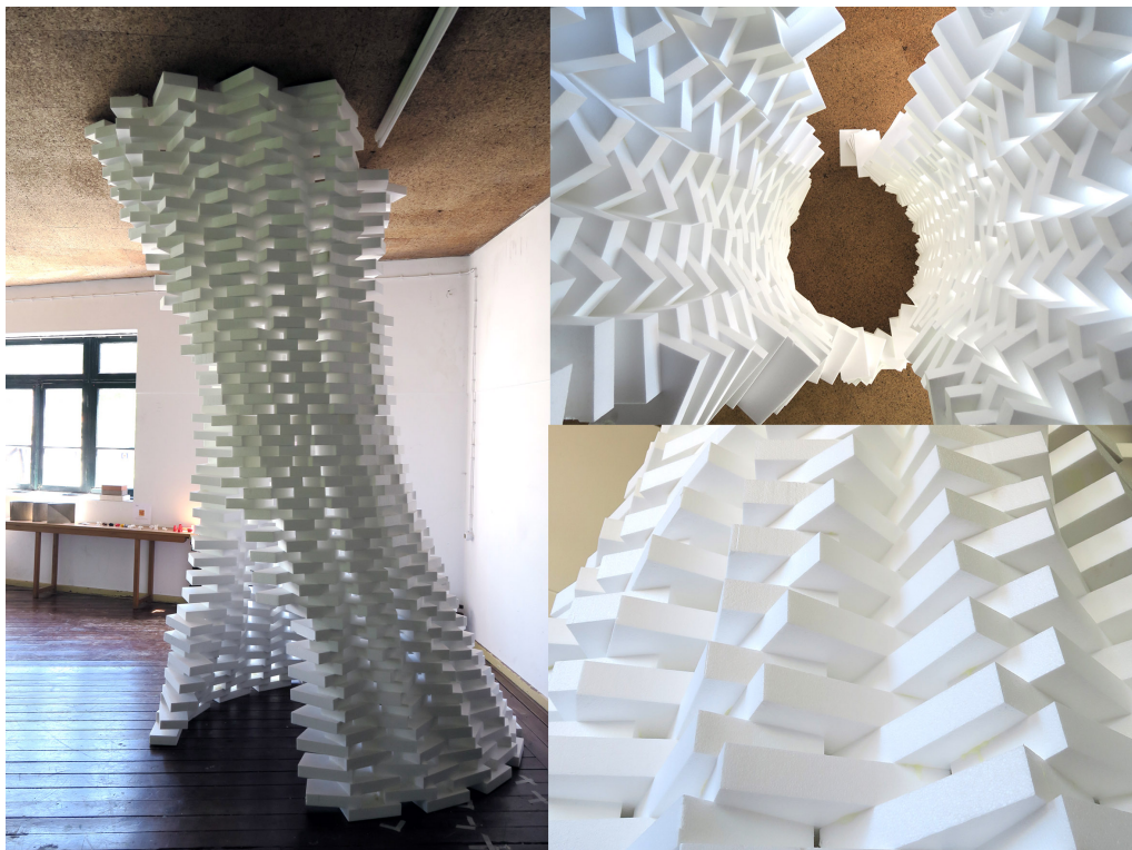
Figure 8 The Brick Tower structure made out of the 2 fabricated parts. On the right, detailed views from the interior (top) and the exterior (bottom).
