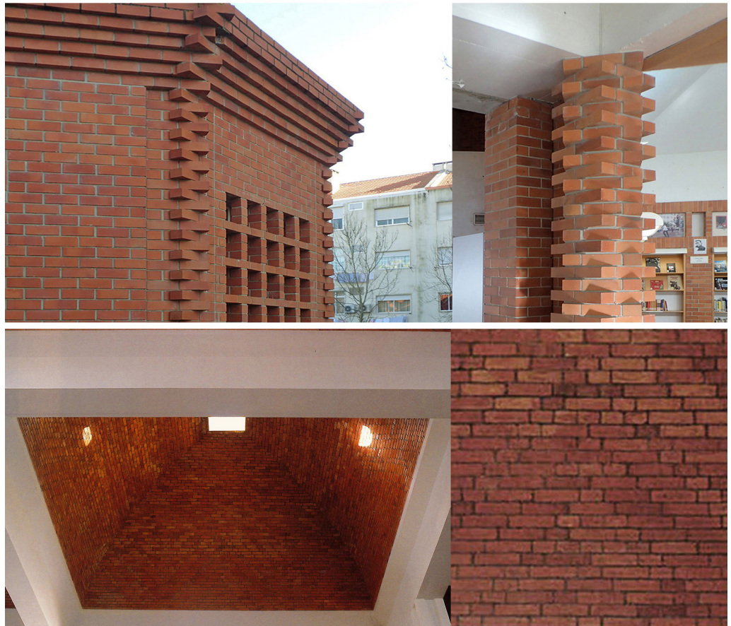
Figure 1 Brickwork details of a column and a corner in the Municipal Library building in Moita (top). One of the domes in the House of Culture in Beja and the detail of its brickwork, which was specifically designed for structural purposes (bottom).
