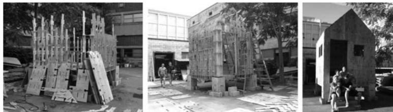
◀ Figure 9: Sequence of assembly starting with the waffled plywood slab concluding with a full sandwich of plywood sheathing inside and outside with plywood stud structure.
