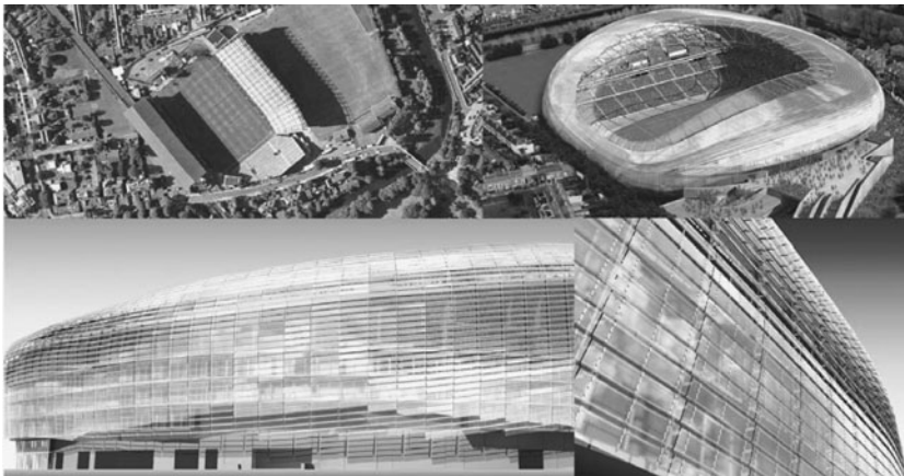
◀ Figure 1. Top left: Site. Top right: Proposed stadium. Bottom left: Proposed façade. Bottom right: Proposed façade detail.
