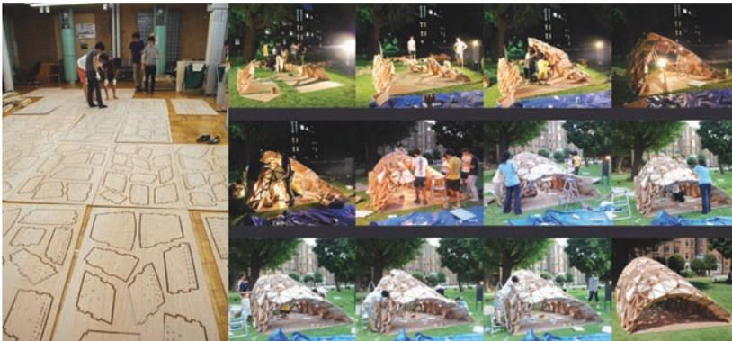
◀ Figure 7: Plywood panels ready for assembly (left), assembly process (right).
