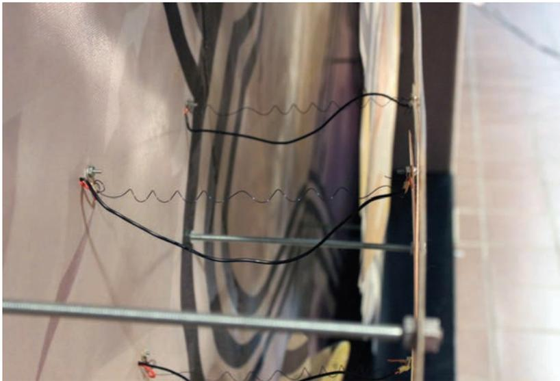
◀ Figure 12: SMA coils attached to the back of the panels.
