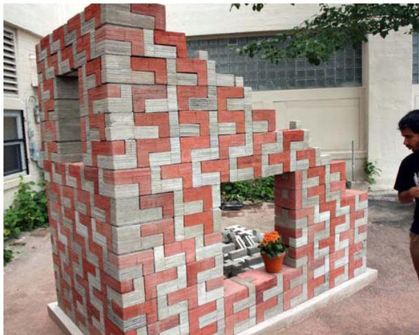
Figure 11. Full-scale corner wall mockup.
