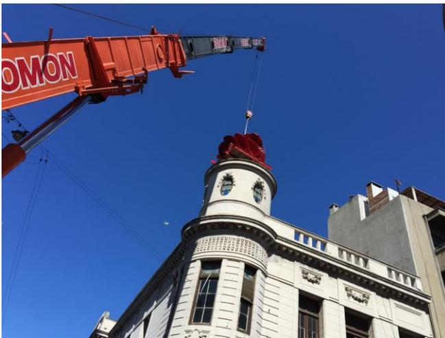
**Figure 3:** Mounting the dome in site.
