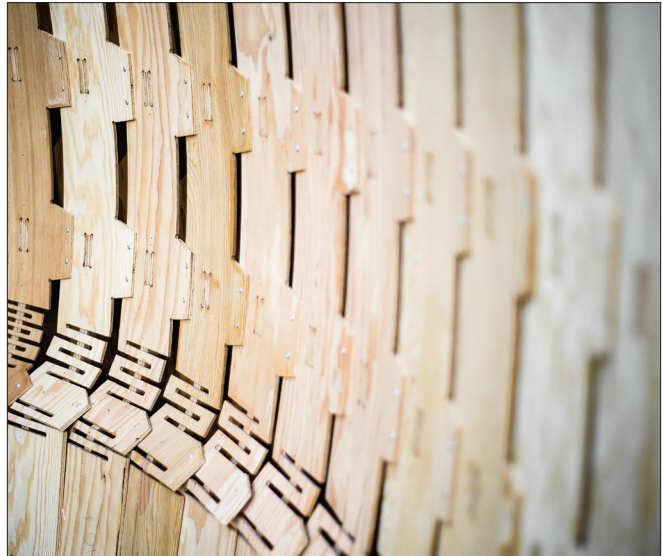
7 Detail of the connections between elements; the stressed skin is formed by vertical plywood strips that connect to each other with flaps, making it possible to bend in a direction other than the strips themselves
