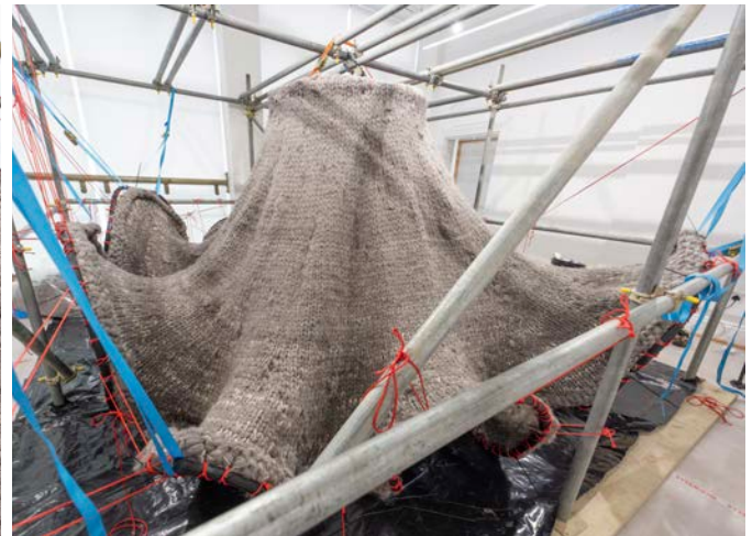
6 Specification for freehand knitted canopy formwork extracted from computational model. Image Credit: Jane Scott.
