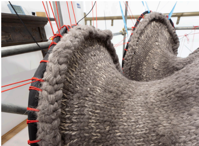
6 Specification for freehand knitted canopy formwork extracted from computational model. Image Credit: Jane Scott.
